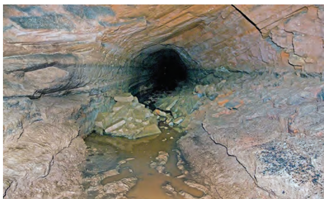
Some distance into the tunnel is this very wide area. Was this a place where boats could pass, an erosion point, or where 2 headings met? There was evidence of material falling from the roof - but it was covered in silt and not fresh. Note: the speckles on the floor on the right are bat droppings
